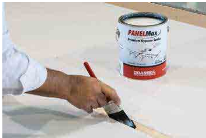
Prime and seal exposed gypsum using PanelMax primer
