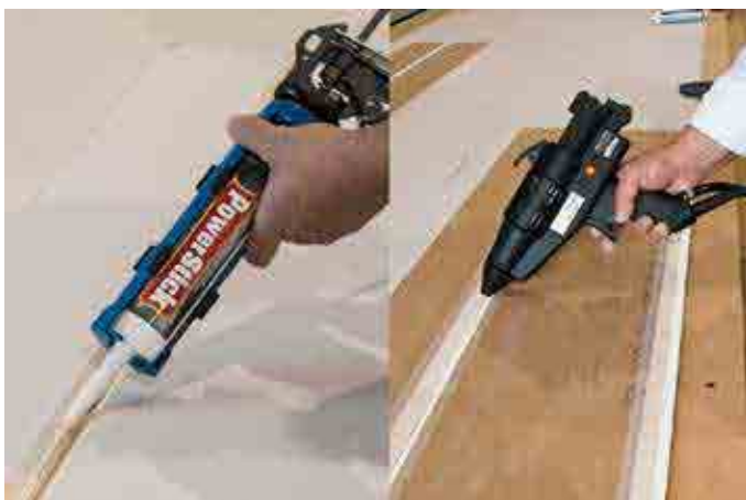
Apply PanelMax hot glue or PowerStick adhesive
